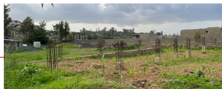
Adwa - Foundations of the main building and walls around the property
