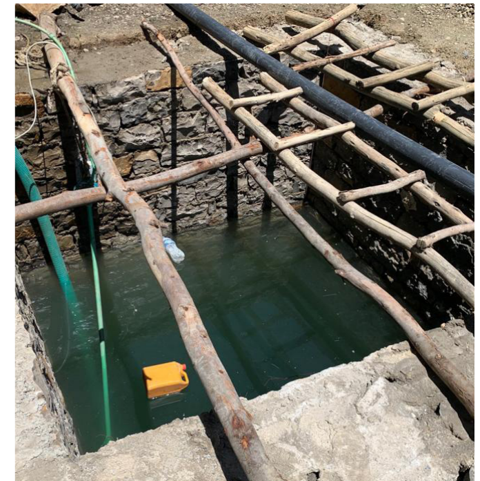
The new shallow well
